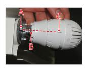
2) Connect the thermostatic head to the valve, making sure the valve pin (A), the small slot on the thermostatic head (B) and the indicator line (C) are aligned.
